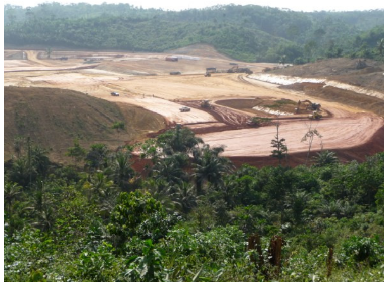
Plant Site Well Advanced
